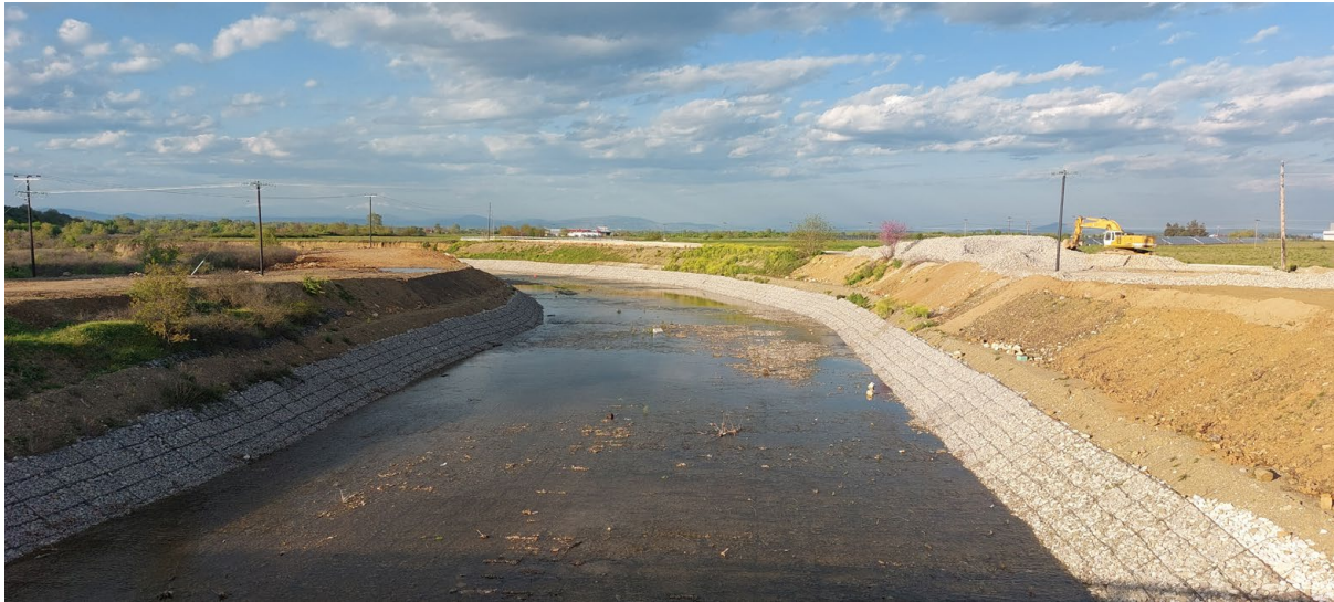
Figure 1. Grey infrastructure situation with dams and gabions along the Kalentzis river
